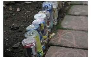
To build the eco-brick wall.
